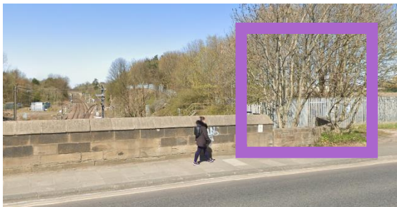
Figure 15 Rail Substation on Whitley Road
